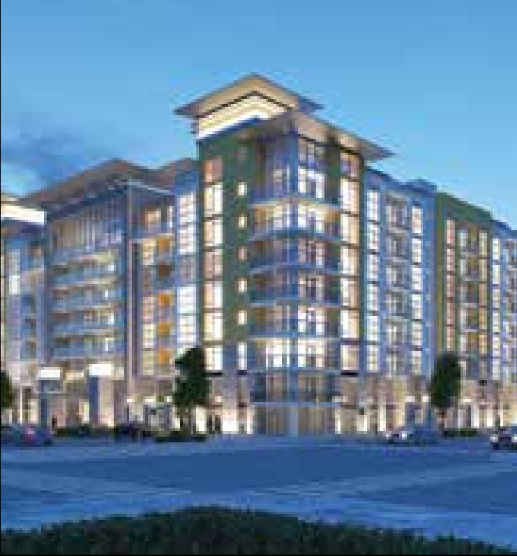
THE HERMITAGE APARTMENT HOMES™, ST. PETERSBURG
